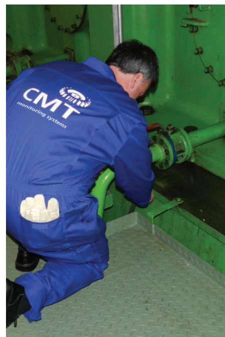
Taking a cylinder drain oil sample from the scavenge space.
